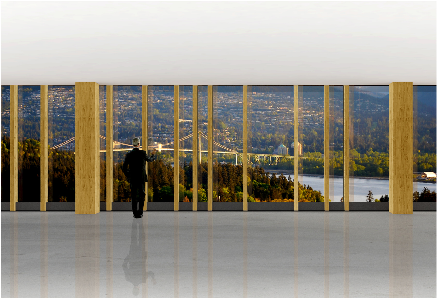
Interior perspective illustrating a glulam curtain wall
